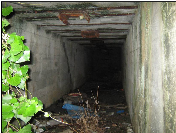
Plate 3 – Showing One of the Tunnels on New England Hill
