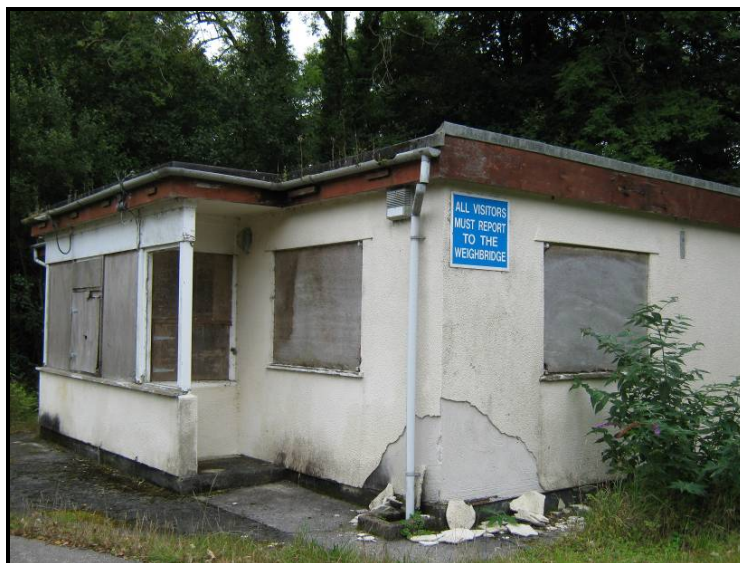
Plate 2 – Building G (Reported to Support a Common Pipistrelle Maternity Roost)
